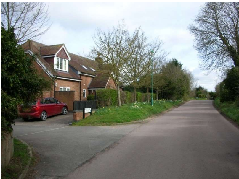
Figure 6.6 As development approaches the settlement boundary the housing density falls considerably (Ashwell Street/ Moules Yard)
