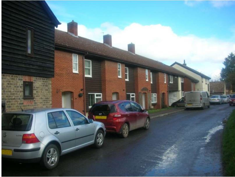
Figure 6.2 The Bear Farm housing development and the scale of the houses themselves reflect the character of their surroundings, in this case in a high-density part of the village characterised by short terraces containing small numbers of dwellings (Bear Lane/Back Street)
