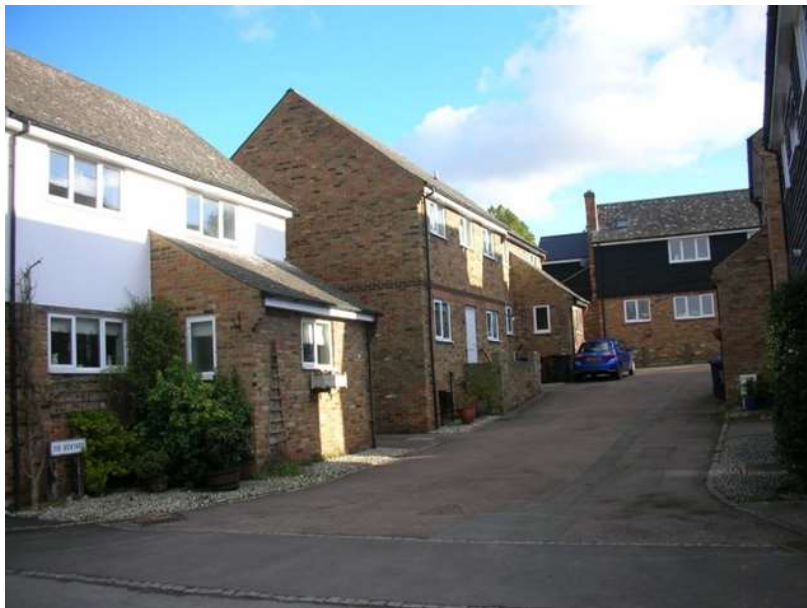
Figure 6.3 The Rickyard is a courtyard style and not a sprawling Close-style development. It is in keeping with its surroundings yet still provides adequate parking spaces
